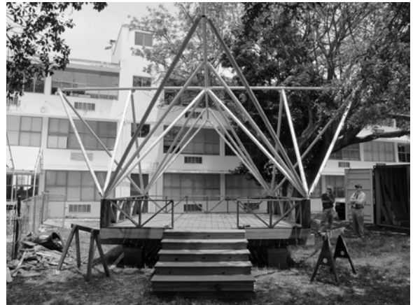
Figure 7: Framing and platform for Eco-tent with the canvas removed.
