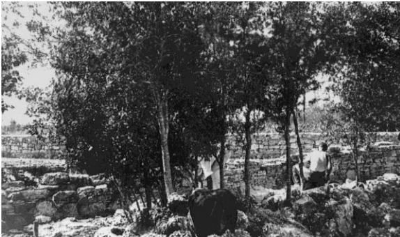
Matheson Hammock Firebreak wall 1935, courtesy of the National Archives
